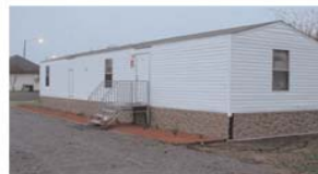
Leonville Utilities Office
