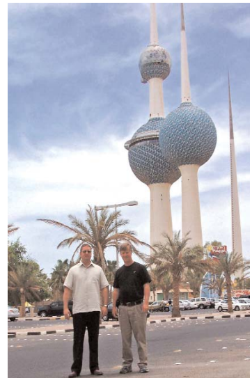
The three towers were built for multi-purpose operations. The needle shaped tower provides electricity to the suburbs in Kuwait. One tower stores up to one million gallons of water. The towers were damaged heavily by the Iraqis during their occupation of Kuwait from 1990 to 1991.
